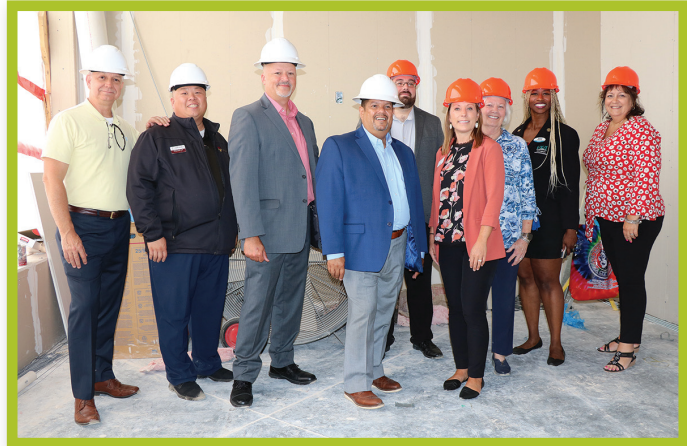
Julio Rodriguez tours the new SIMMS construction site. Left to Right: Steven Mitchell, Economic Development Director, City of Carbondale; William Lo, Executive Director, Carbondale Chamber of Commerce & IWIB Member; Bryan Ellis, Downstate Workforce Development Regional Manager, DCEO; Julio Rodriguez, Deputy Director, Office of Employment & Training, DCEO; Jordan McBride, Program Manager, Man-Tra-Con; Emily Perks, Employer Services Manager, Man-Tra-Con; Mary Roe, Man-Tra-Con Corporate Board President & Southern Illinois Workforce Development Board Vice-Chair; Tamiko Mueller, Jackson County Chief Local Elected Official; Robyn Russell, CEO, Man-Tra-Con.
